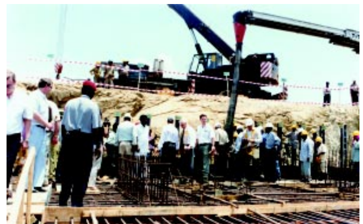
Ground Reality : The Project work at Kudankulam begins with a bang.
