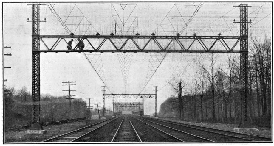
Each catenary consists of two 1/2-inch steel cables carried on insulators on the top of the trusses. The copper trolley wire is suspended from the cables and held in level and alignment by triangles made of 3/2-inch pipe.
