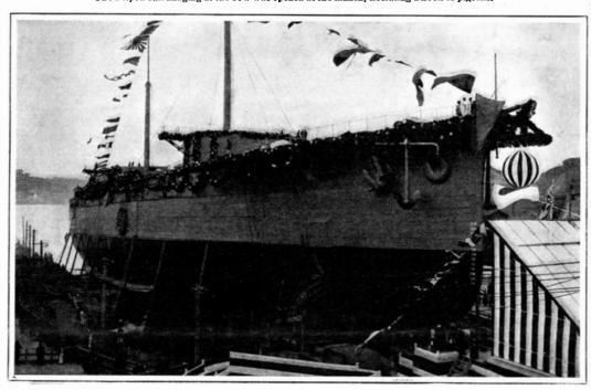
Length, 482 feet. Beam, 83½ feet. Displacement, 19,200 tons. Horse-power, 18,000. Speed, 20 knots. Armor: Belt, 9½ inches. Armament: Four 45-caliber 12-inch; twelve 45-caliber 10-inch; twelve 50-caliber 4.7-inch. Torpedo tubes, 5.
