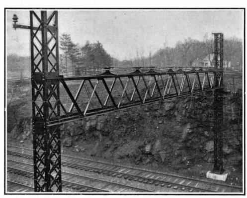
Near View of Steel Posts and Truss, Showing Method of Attaching Catenaries.
