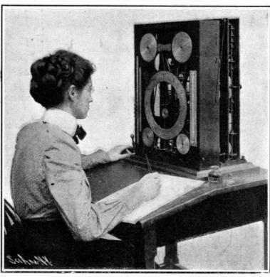
Operator Turning Indices to Determine the Height and Time of the Tide at a Future Date.
