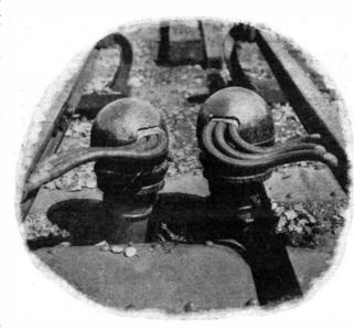
Third-Rail Jumper Connections Used at Cross-Overs.
